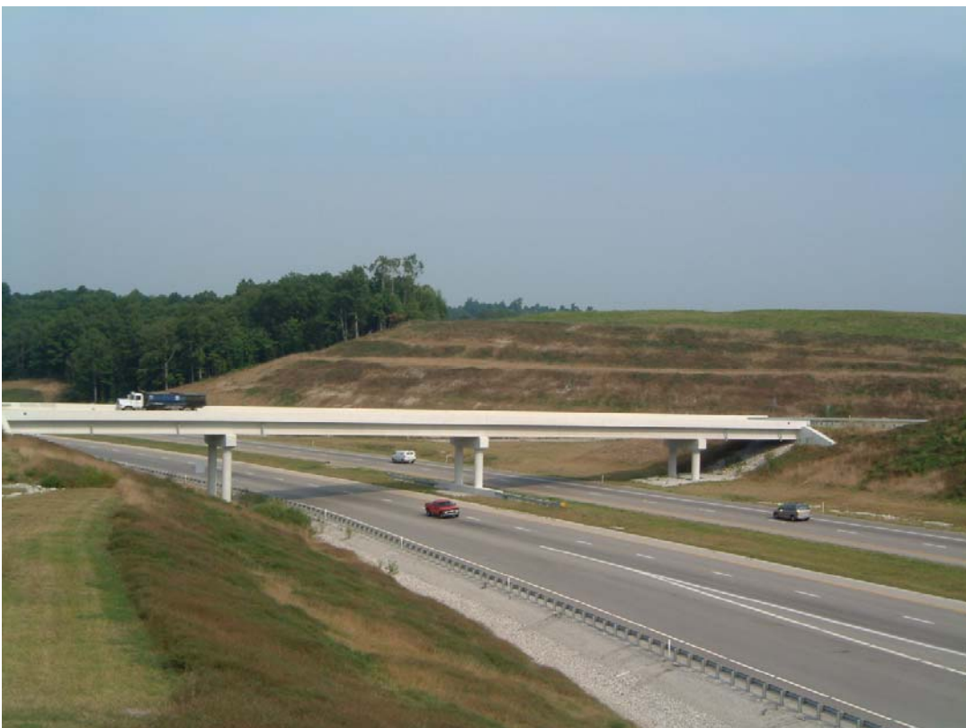
Industrial Parkway Over I-64
